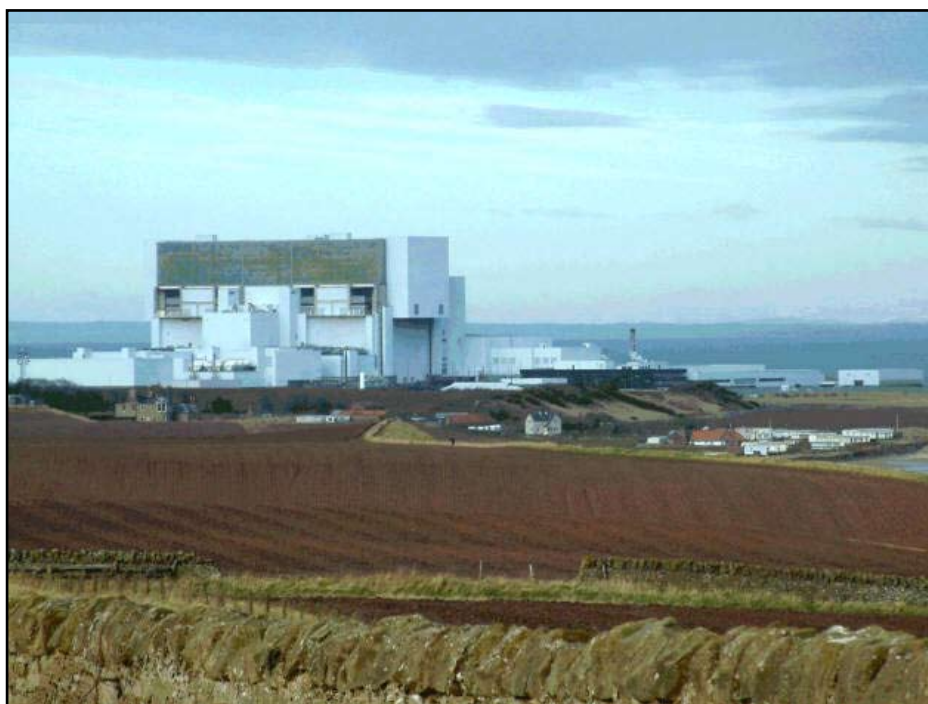
Torness Nuclear Power Station, East Lothian
