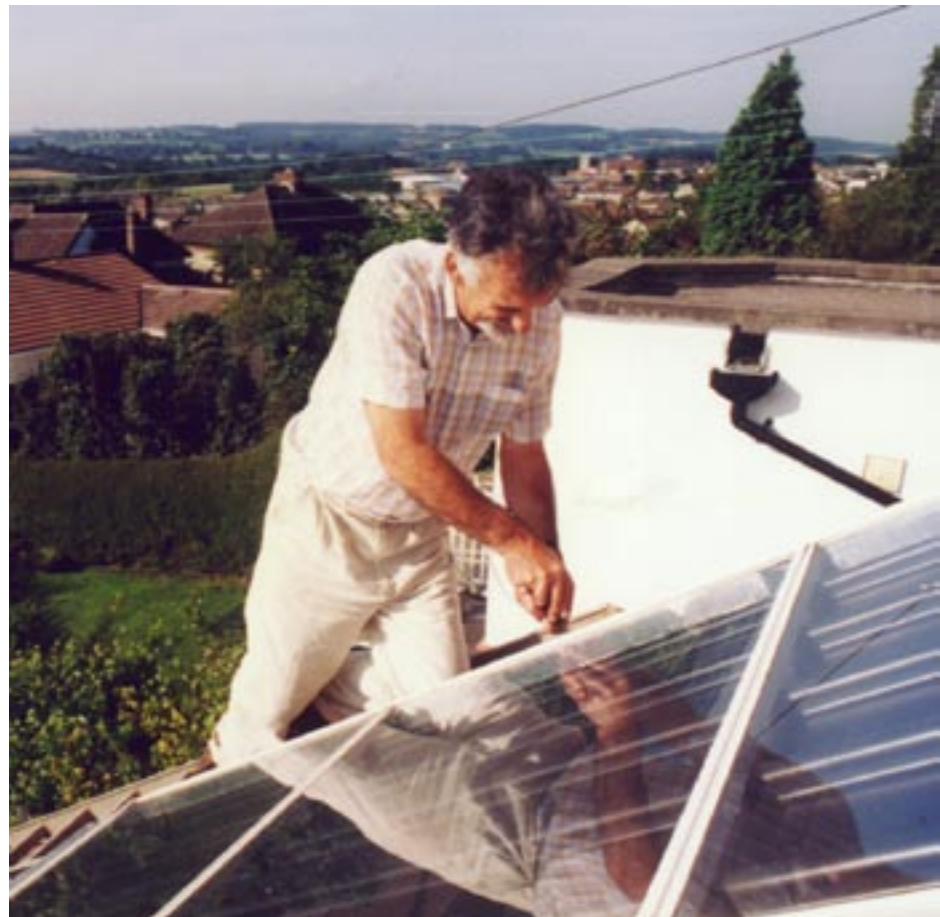
Householder fitting Solar Water Panels to his roof.
